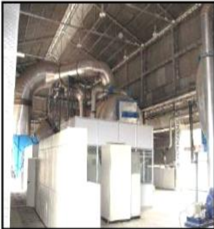
Fig: MVR type Evaporator System installed in all CETPs
