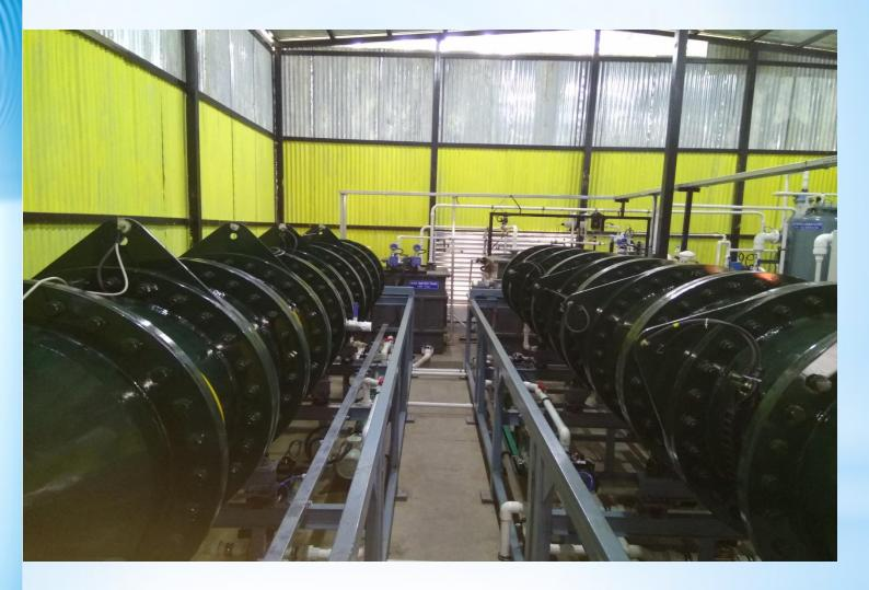
150 KLD expandable to 600 KLD, FPSTAR system Installed in Pune, India, Processing Food Industry Effluent to drinking grade water for Reuse..
