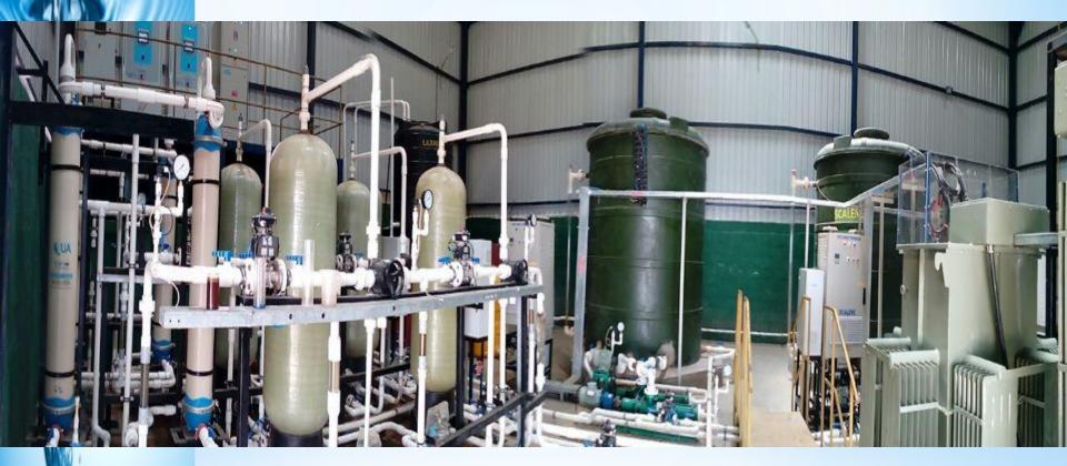
400 KLD, FPSTAR system Installed in Karnataka, India Processing Coffee Pulping Effluent for complete Reuse..
