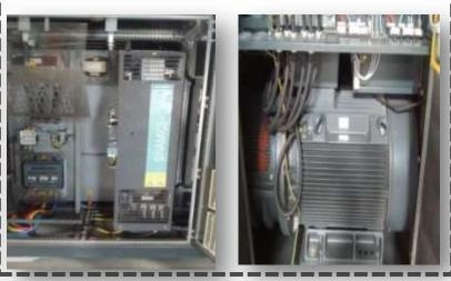
VFD INSTALLATION FOR COMPRESSOR
