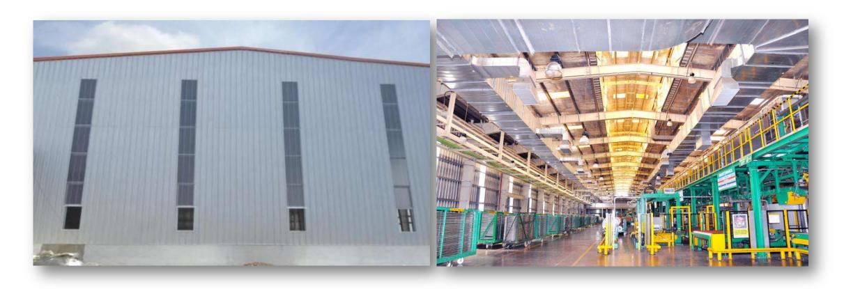
Maximum utilization of Day light as a substitution of Electrical light in day time by installing transparent acrylic sheets.
