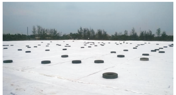
5 th CELL UNDER CONSTRUCTION
